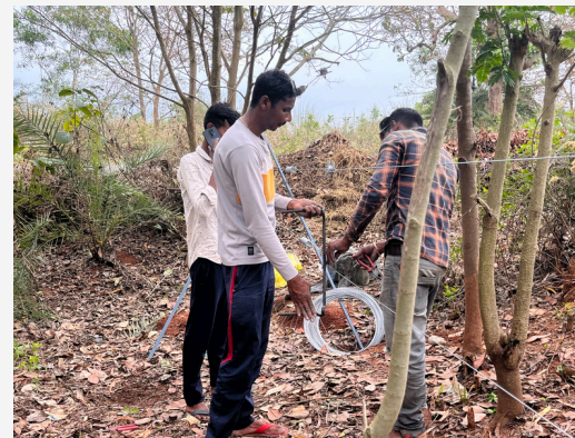
Installation work in progress in Choto Kuraria
