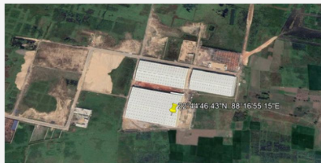
Encroachments at Joykrishnapur, Dankuni ②
