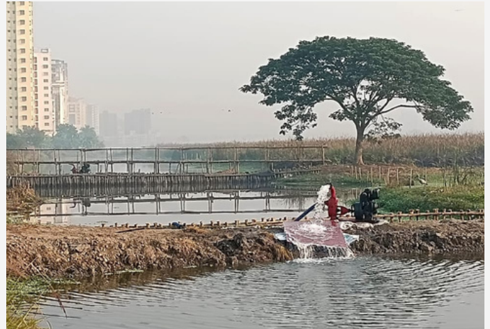
The bridge under construction at the site of encroachment
